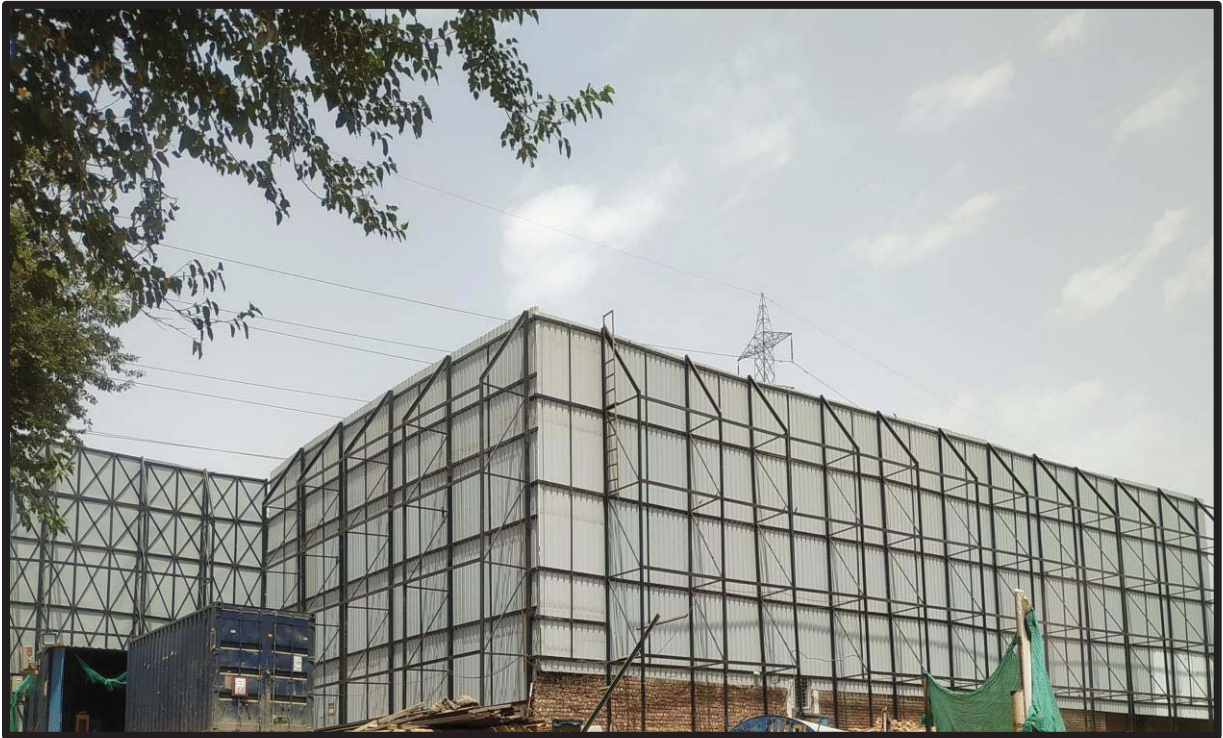
Front - Inside Barricading
